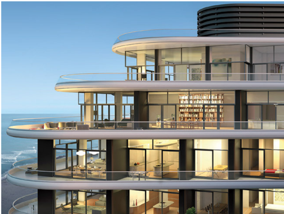
Terraces at Faena House.
